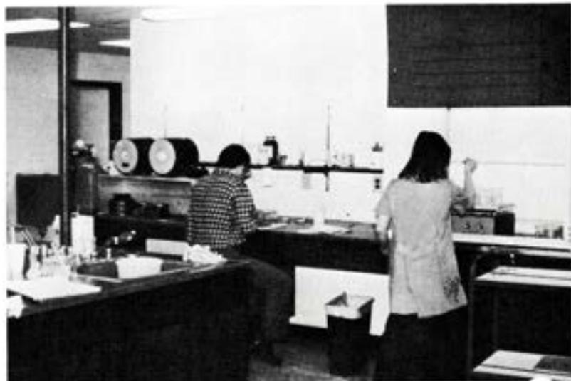
General laboratory view showing two fusion furnaces and laboratory hood.
