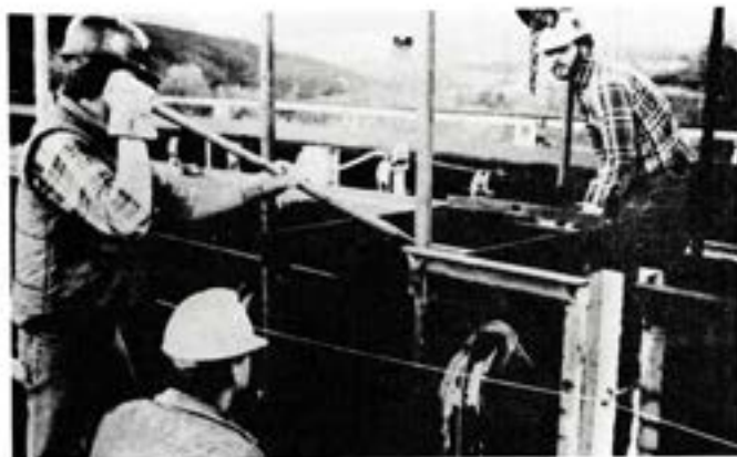
Above, crushing the gross sample and subsequent subdivision by riffling.
