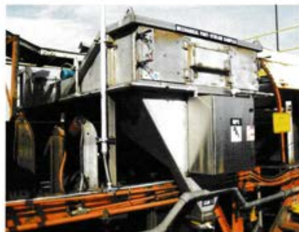
Figure 2. Installation of a Mechanical Part-stream Sampler (MPS).
