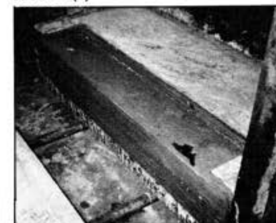
Floor plate readied for higher temperature castable (8)
