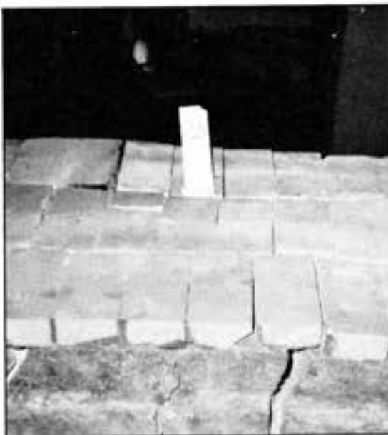
Old brick up to tier 23 indicating the deterioration of refractories (3)
