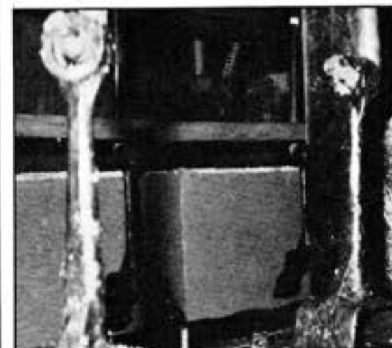
Stainless steel greased hanger for suspension of the arch (7)
