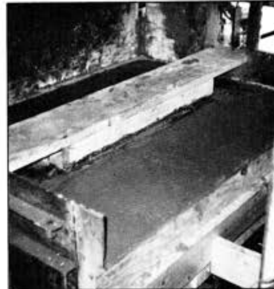
Wooden forms used to contain high temperature (4) castable material (Tiers 1-4)
