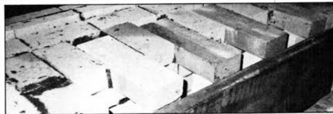
Kicker brick for support of wall plates (6)
