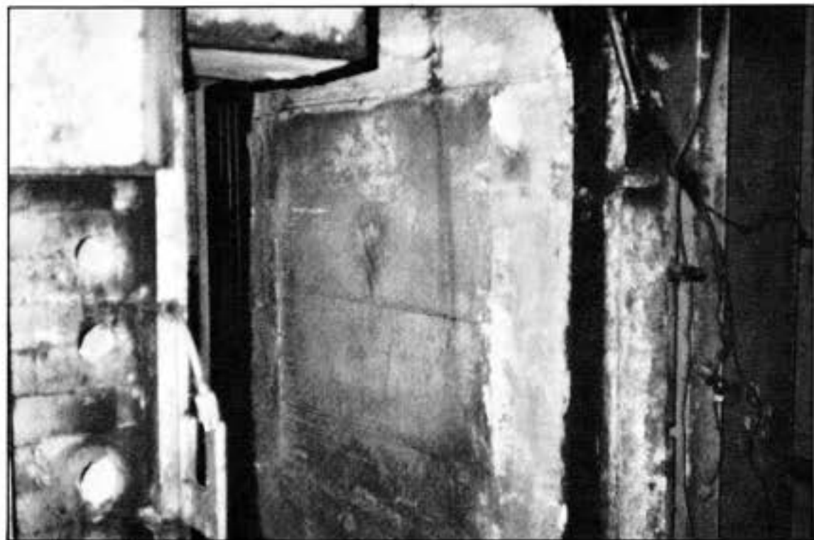
Movable wall of oven before rebuild (1)
